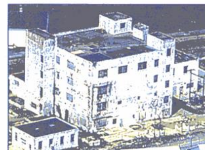
Former CW Production Facilities
